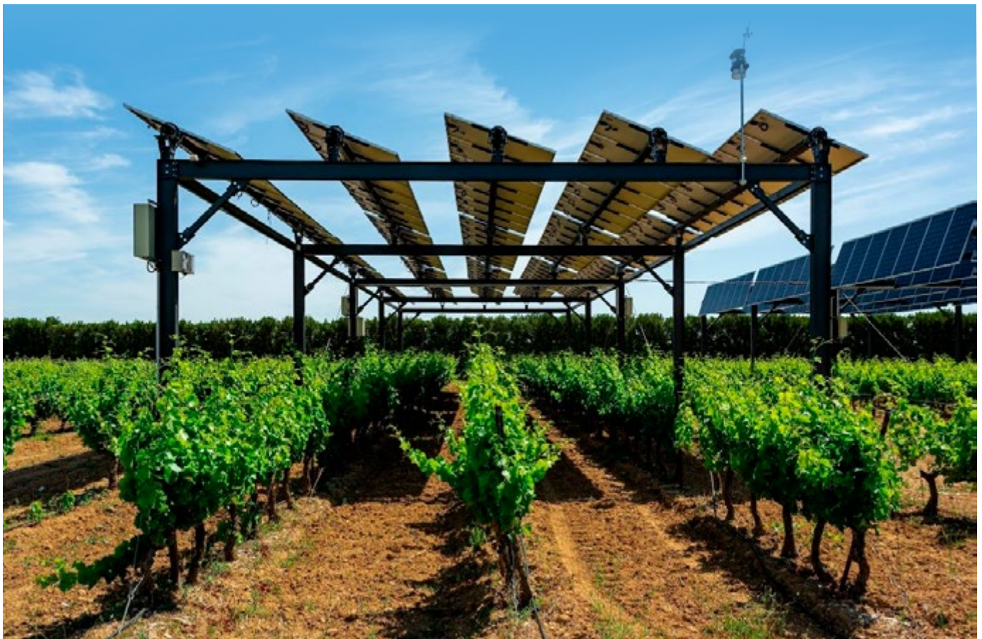
Figure 3 Movable panels over grapes in Piolenc, southern France (photo: Sun'Agri 8 )
